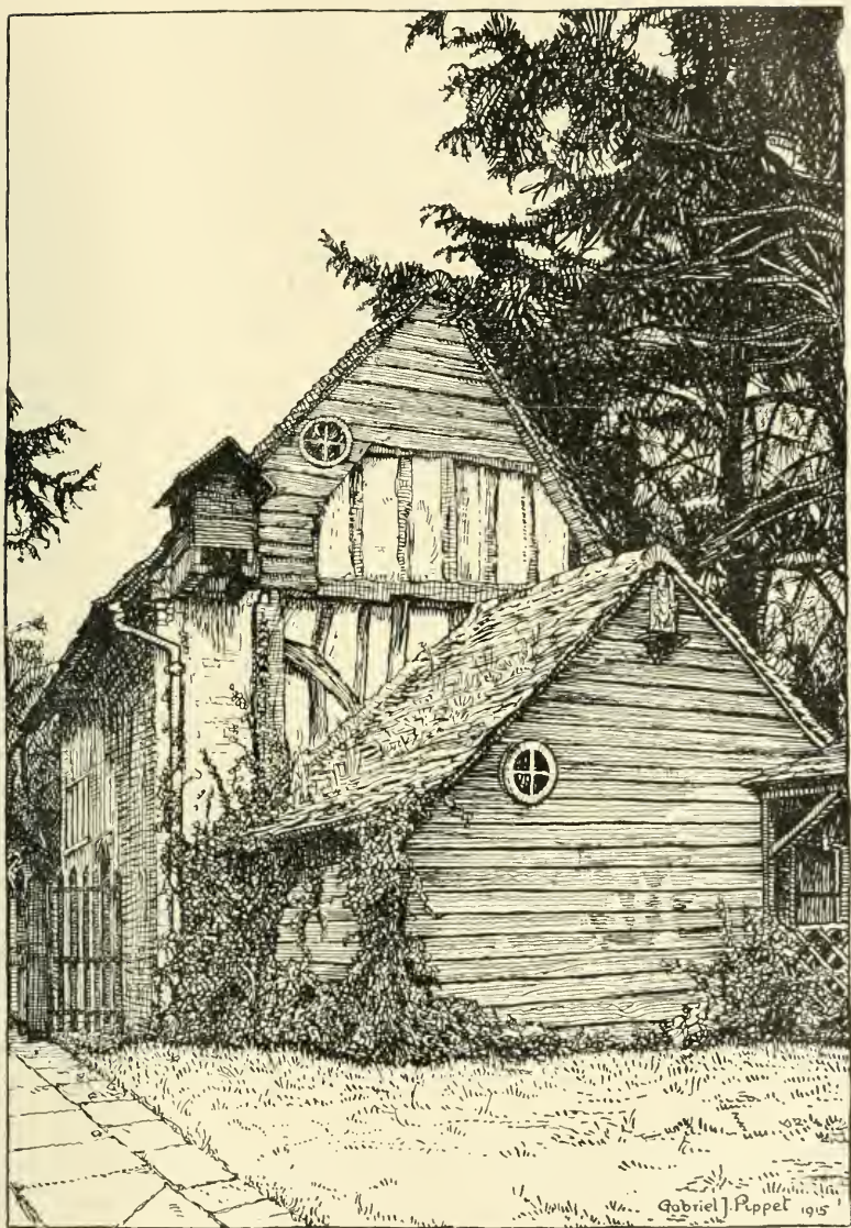
HARE STREET CHAPEL: EXTERIOR
